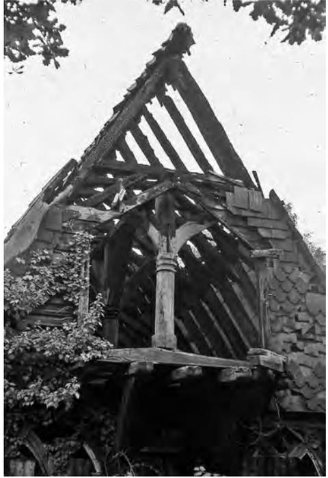
*Hall roof after fire damage, revealing tie beam and crown post.*
