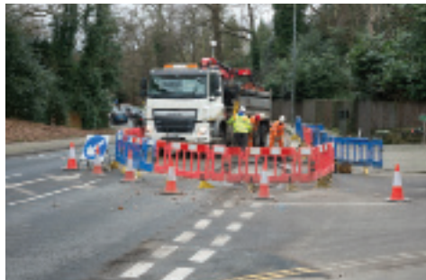
LBB now provide us with information on emergency road works
